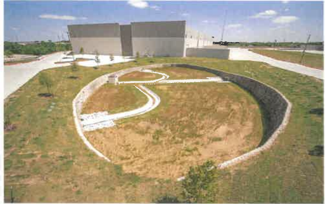
Retention ponds can help manage stormwater runoff by collecting and storing excess rainwater, reducing the risk of flooding. It also improves water quality by allowing sediments and pollutants to settle before the water is released into the environment.
