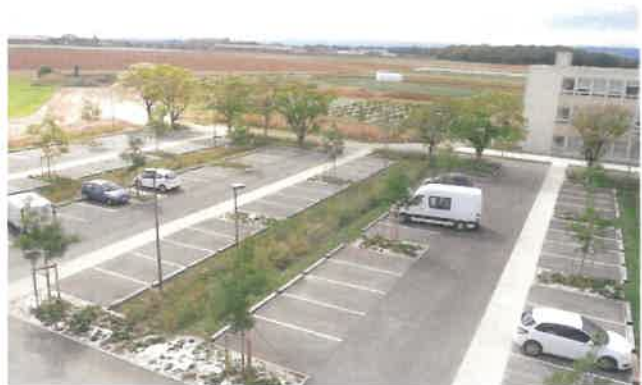
Surface parking areas allow parking for a mix of utility trucks, workers and visitors alike. They also allow for the use of more pervious materials and other low-impact development techniques.
